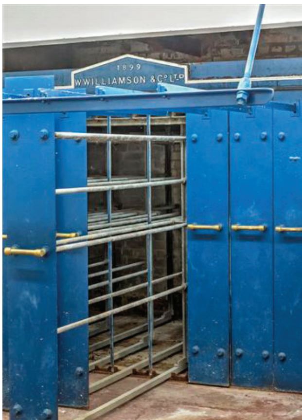
Fig. 2: The drying closet has nine vertical sets of clothes horses with brass handles that slide in and out of the closet. Steam from the boiler room was fed into a calorifier (heat exchanger) above the closet. Air was blown over the pipes inside the calorifier by a fan, driven by the steam engine via the driveshaft.
