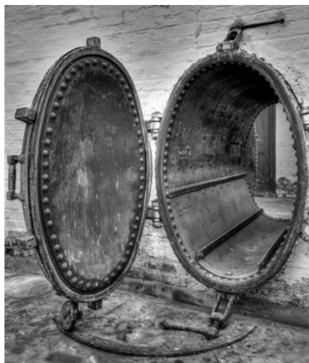
Fig. 4: Autoclave for the disinfection of linen using formalin. It is built into the dividing wall between the room where soiled linen was loaded and the room where the disinfected linen was extracted and taken to be washed, dried and ironed. The linen was held in a deep, metal-framed wire-mesh basket with a high handle with a cross-bar and hooks from which it could be suspended. The basket slid in and out of the autoclave on four wheels that ran on a track inside the machine. Note the heavy doors and the handles to prevent leaking.
