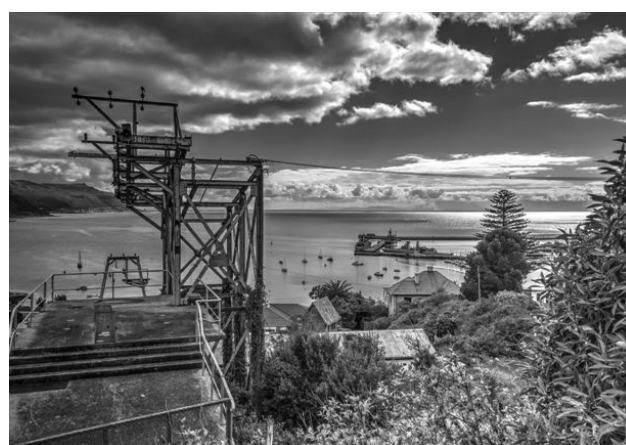
Fig. 6: Aerial ropeway lower landing stage, which was the main access to and from the ropeway for the hospital. The ropeway engine room was situated here.
