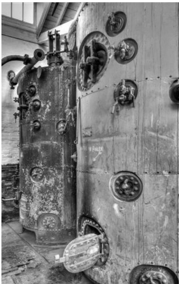
Fig. 5: Vertical boilers of a standard Victorian design used to power a variety of equipment. The vertical design was easier to fire and maintain than a horizontal boiler. Although not particularly efficient, this was not of major concern as coal was cheap. The attendant stoker introduced three to four shovelfuls of coal every half hour or so.
