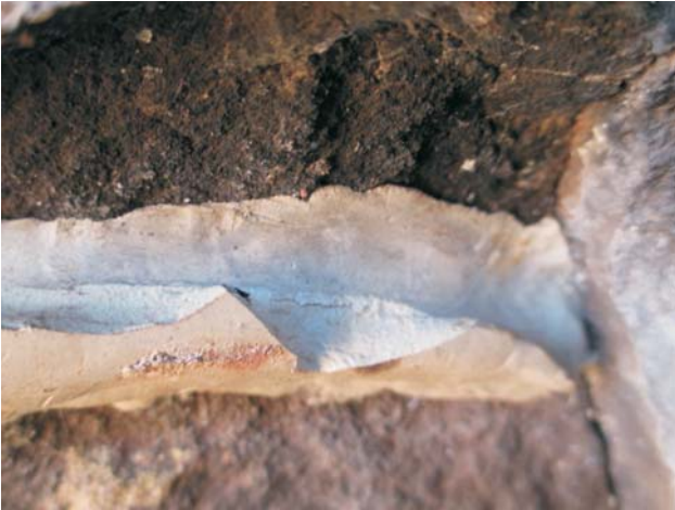
Fig. 4: Vandalism to the dripline at Bhlendleni Shelter, 2014
