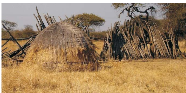
Fig. 2: The gradual decay of the beehive houses. Note the missing thatching grass lower down caused by cattle grazing.
